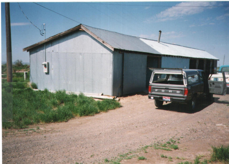
BUILDING HOUSING WELL + PRESSURE TANK
