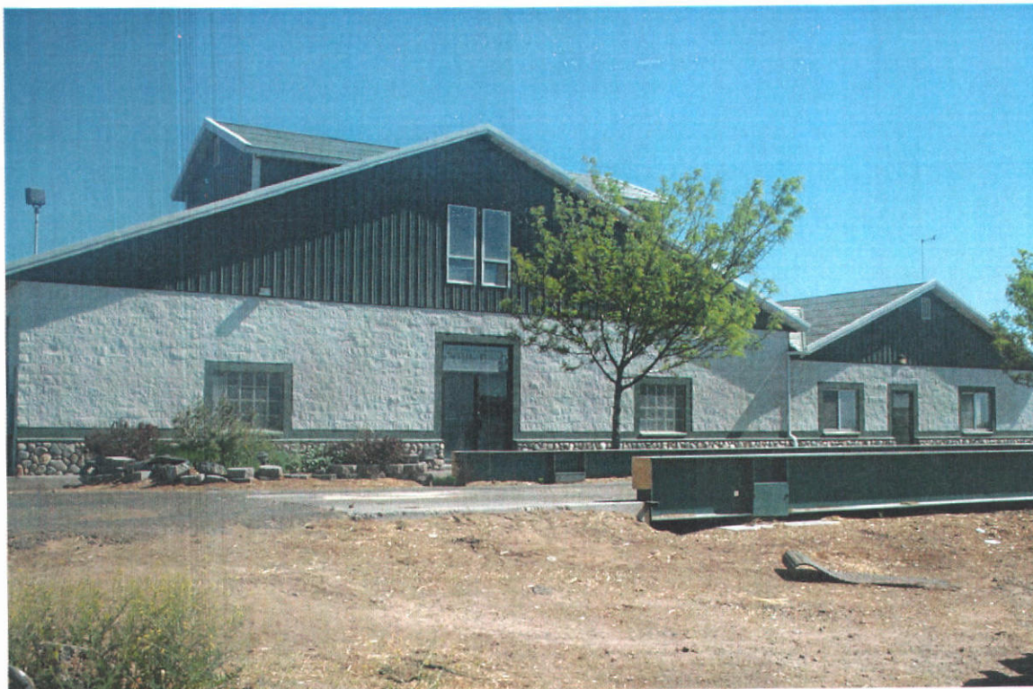
Dairy barn looking NE Wells are in grass strip between the small trees By J E Stanton 5-30-02 Permit 36-8736
