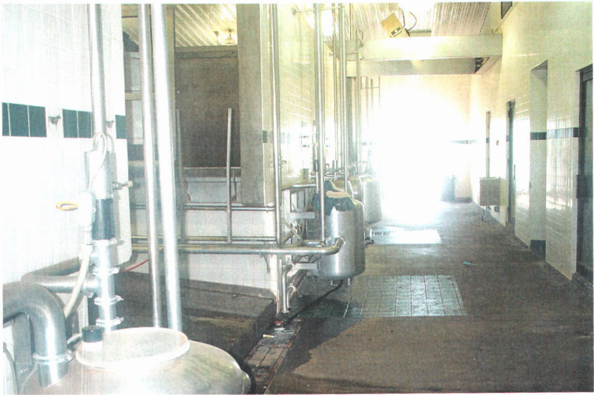
Inside of dairy barn By J E Stanton Permit 36-8736
