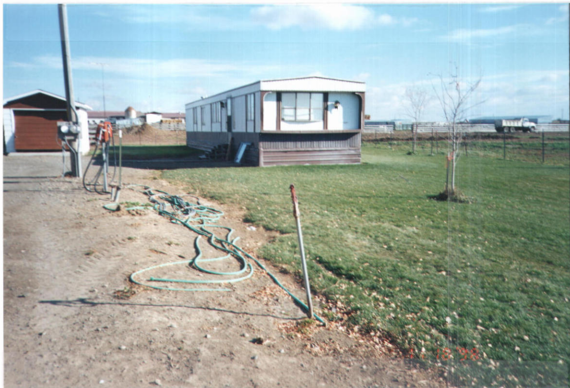
Mobile Home (Well under spigot)
