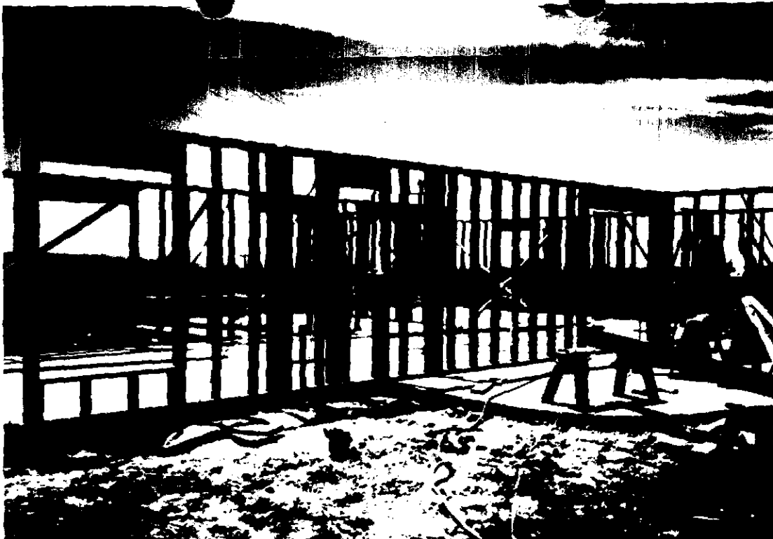
Home Under Construction W of Existing Home
