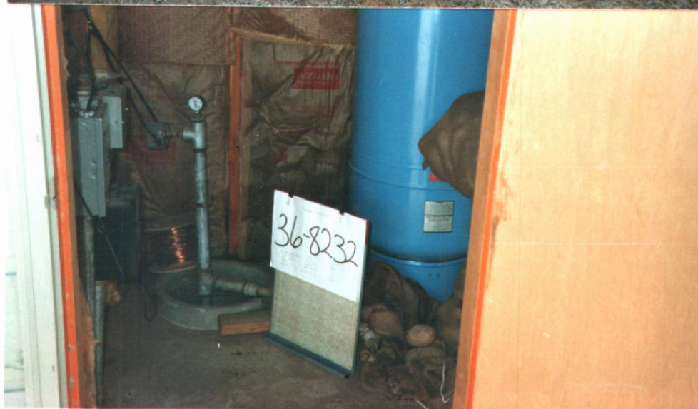
Well House of E. well 2nd pressure tank in the process of being replaced
