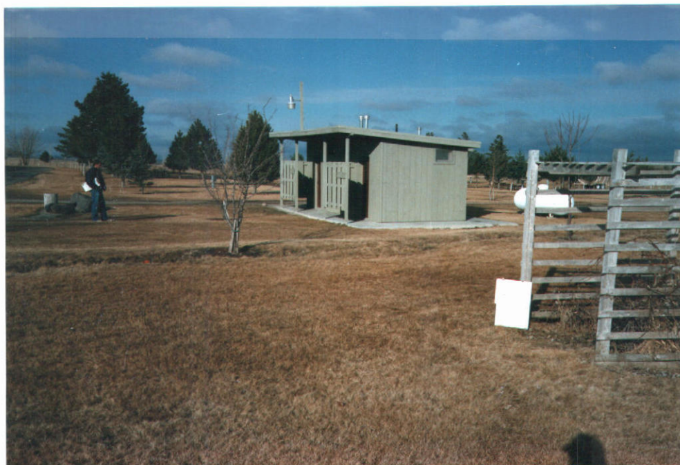
Rest Room in Central R.V. Area
