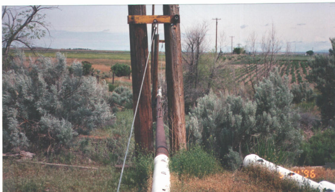
Crossing over creek from South well. (view N)
