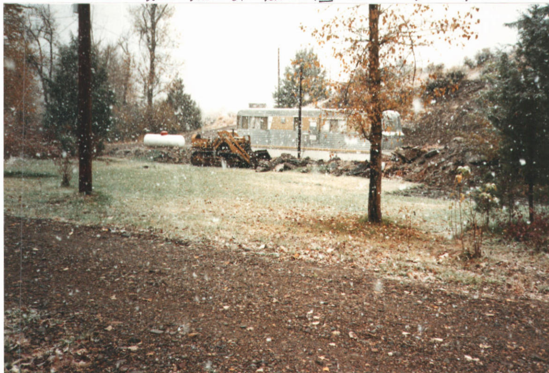
PHOTO FOUR- P/u, closer view of a domestic site with yard.
