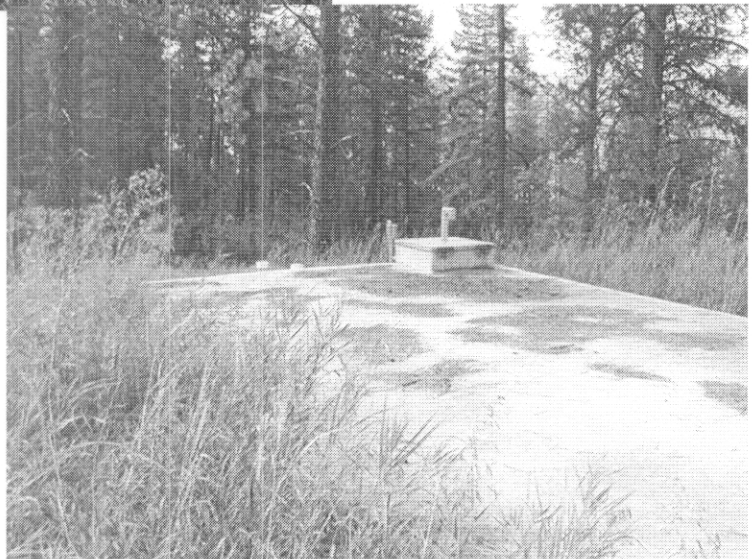
50,000 Gallon Concrete Storage Reservoir (Constructed 1998)
