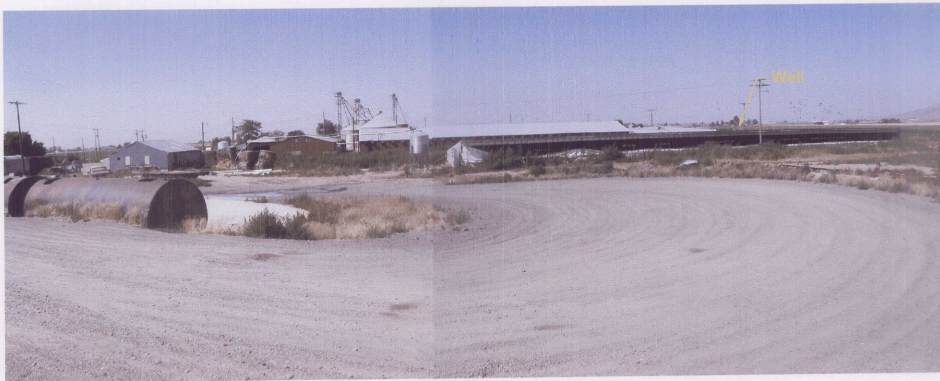
Photo 3: Panorama of facility from south boundary looking north
