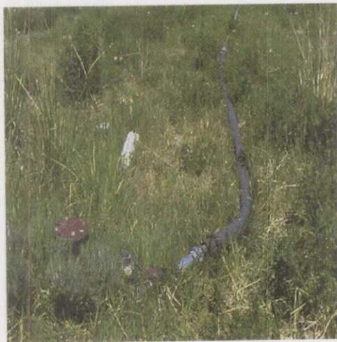
Well and vinyl main line
