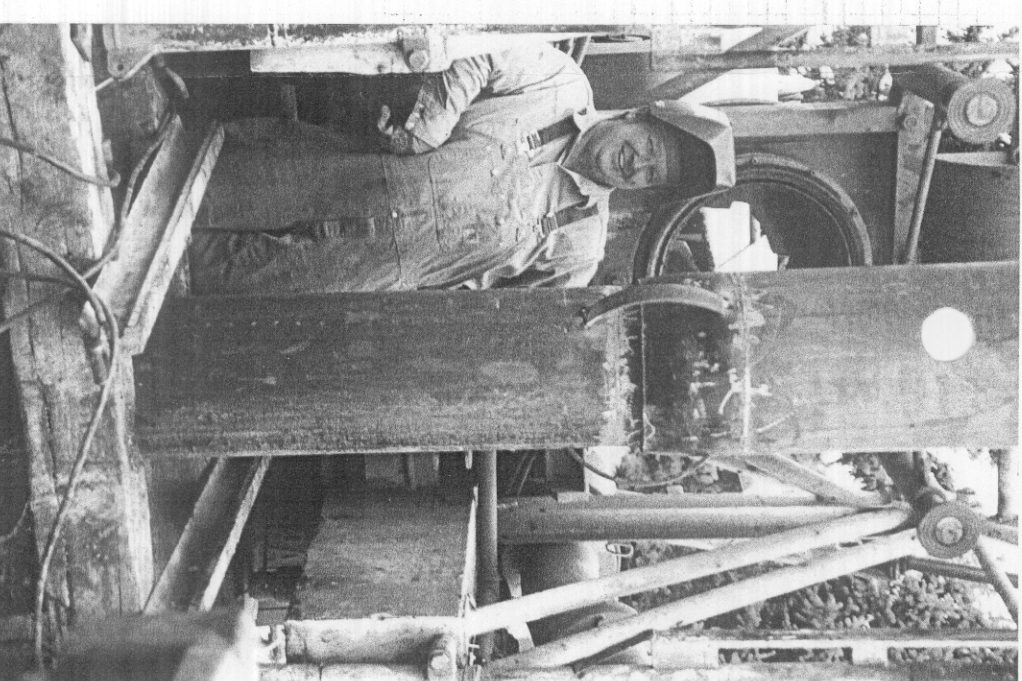
Photograph of the cone-reducer, from the 16-inch surface casing to the 14-inch headpipe and screened liner, during installation of the well casing of the Crane Creek Country Club's Back-9 Irrigation well. Centralizing staves, to ensure a 360° envelope of the filter sand and surface seal as shown straddling the joint.
