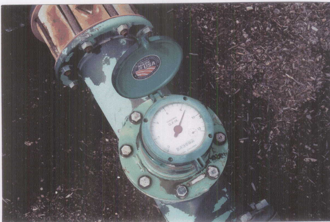
Figure 4. Photographs of the CCCC's Club House Well "Water Specialties" totalizing flow-meter. Upper view shows the serial number of the unit while the lower picture shows the instantaneous diversion rate of 850 gpm and a totalized gallons pumped of 243587 X 1000.
