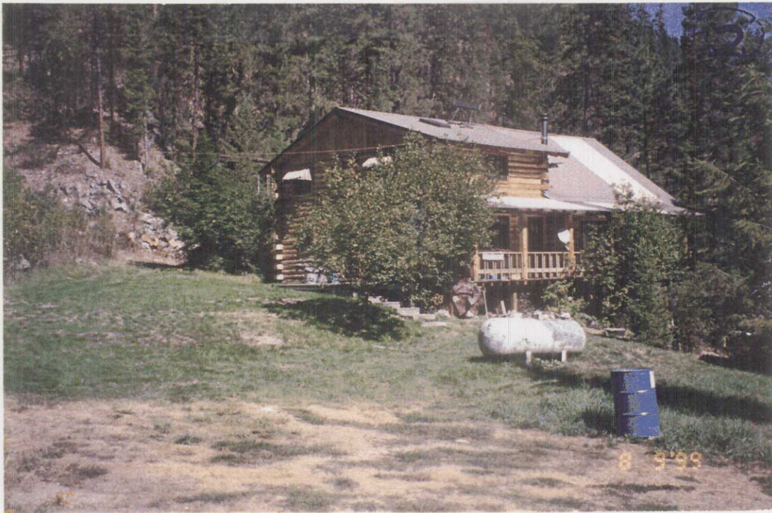
② Cross cabin & yard.
