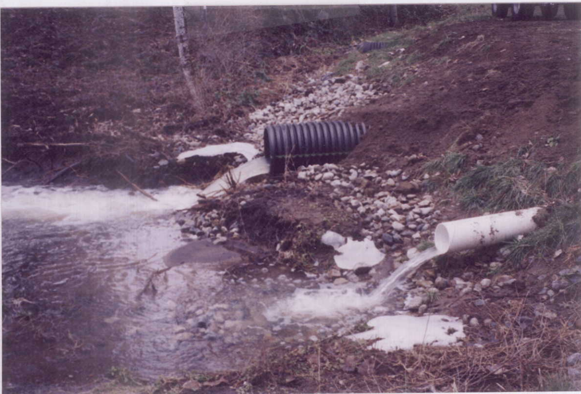
Downstream side of dam.
