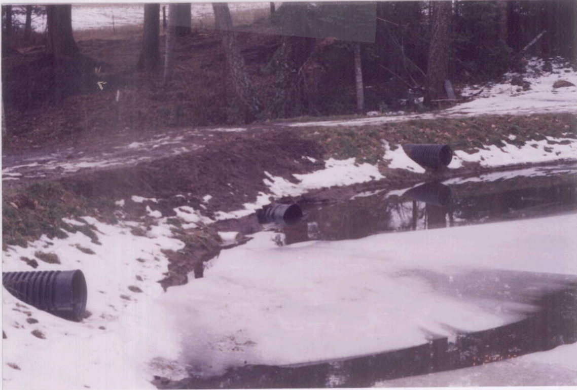
Upstream side of dam showing new outlet pipe (in the middle) installed late last year.
