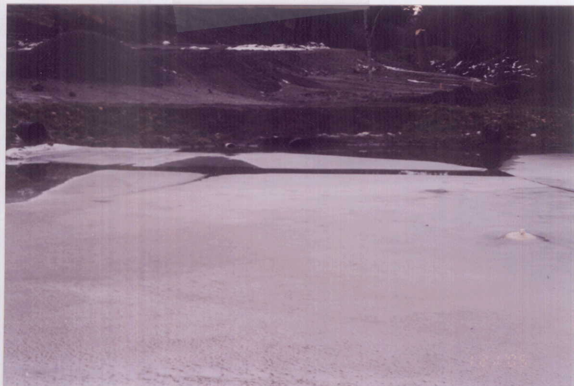
Upstream side of dam at the height of the runoff.
