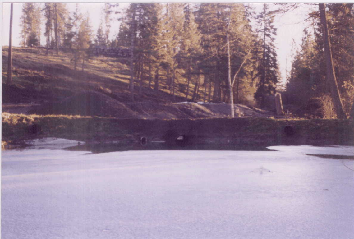
Upstream side of Welburn's dam. The pipe in the middle is new.
