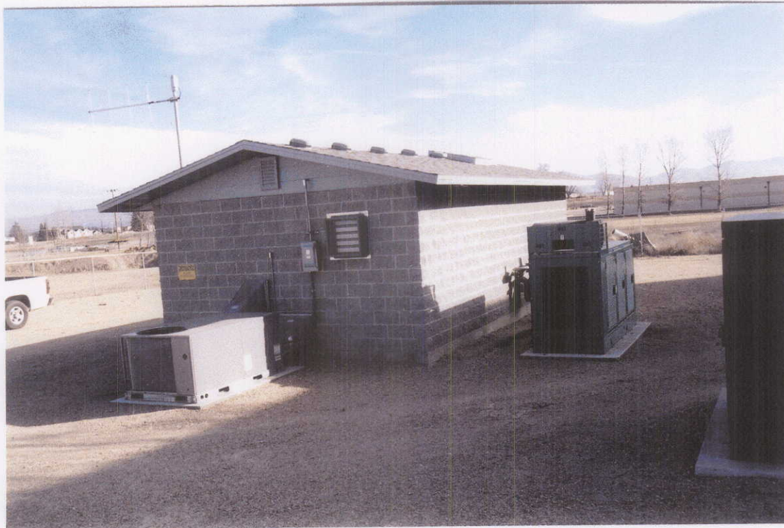
Figure 6. February 11, 2005 photographs of the exterior of the 28' X 16' cinder block Meridian Well #21 pump house at 300 E. Watertower Lane. The upper view looks east at the west and south walls and the lower photo is to the west showing the north and west walls of the structure. Visible in the lower picture is the nearby elevated reservoir to which the Well #21 is pumped. The lower photo shows the back-up natural gas powered generator in case of emergency power outages.
