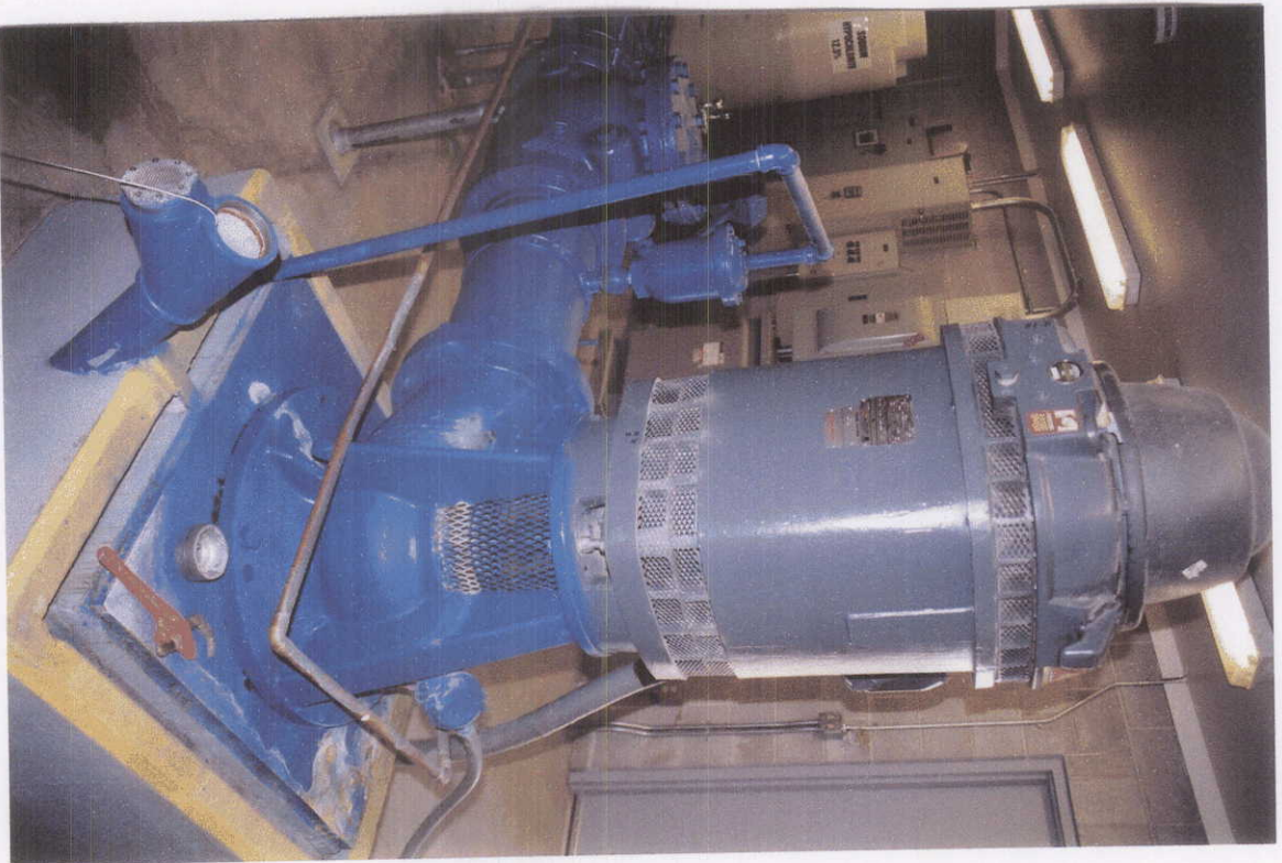
Figure 9. February 11, 2005 photographs of the 125 HP US Motors drive motor for the line-shaft deep well turbine pump installed in the City of Meridian's #21 municipal water supply well. Left view shows the 125 HP motor specification plate and water-level measuring point which is 2 feet above pump house floor. Right hand photo shows the 10-inch discharge head
