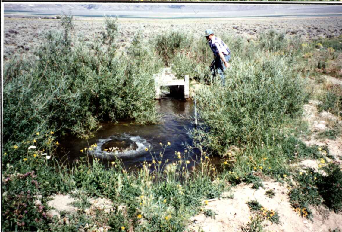
Bubbler & headgate Gravity flow mainline starts at this point & feeds Pivot IN NE 1/4 Sec 15
