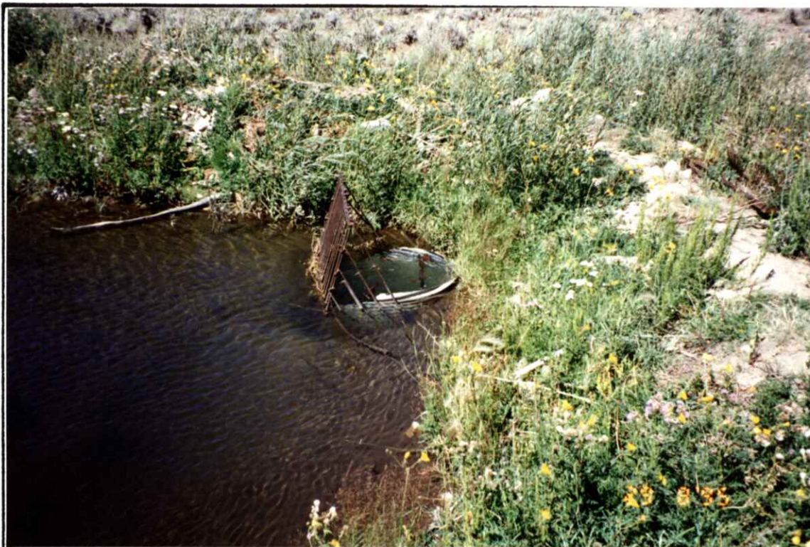
POND & INTAKE SCREEN at Bubbler
