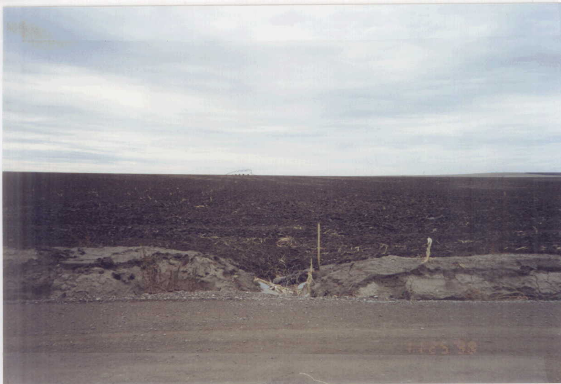
Diversion Works In sec. 14 (looking West)
