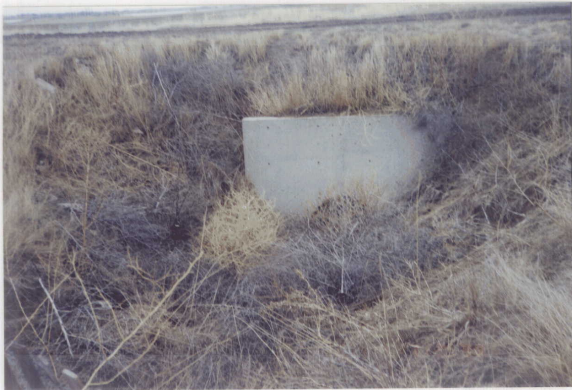
Culvert In Channel Sec. 24 (Looking East)
