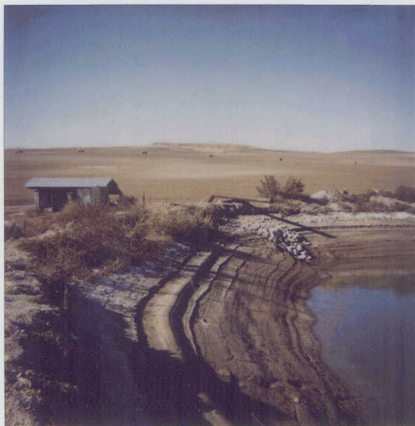
Well, Mainline to Pond
