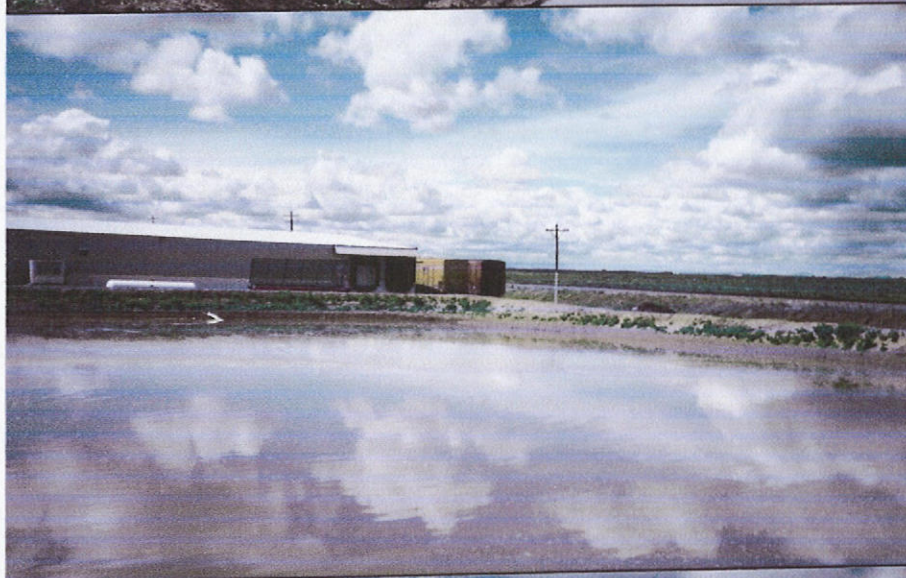
Settling Ponds Looking SW
