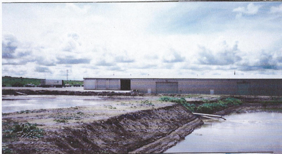
Settling Ponds looking SE
