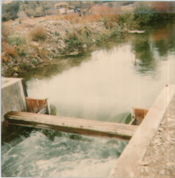
Six foot weir on ditch to the west below the power plant
