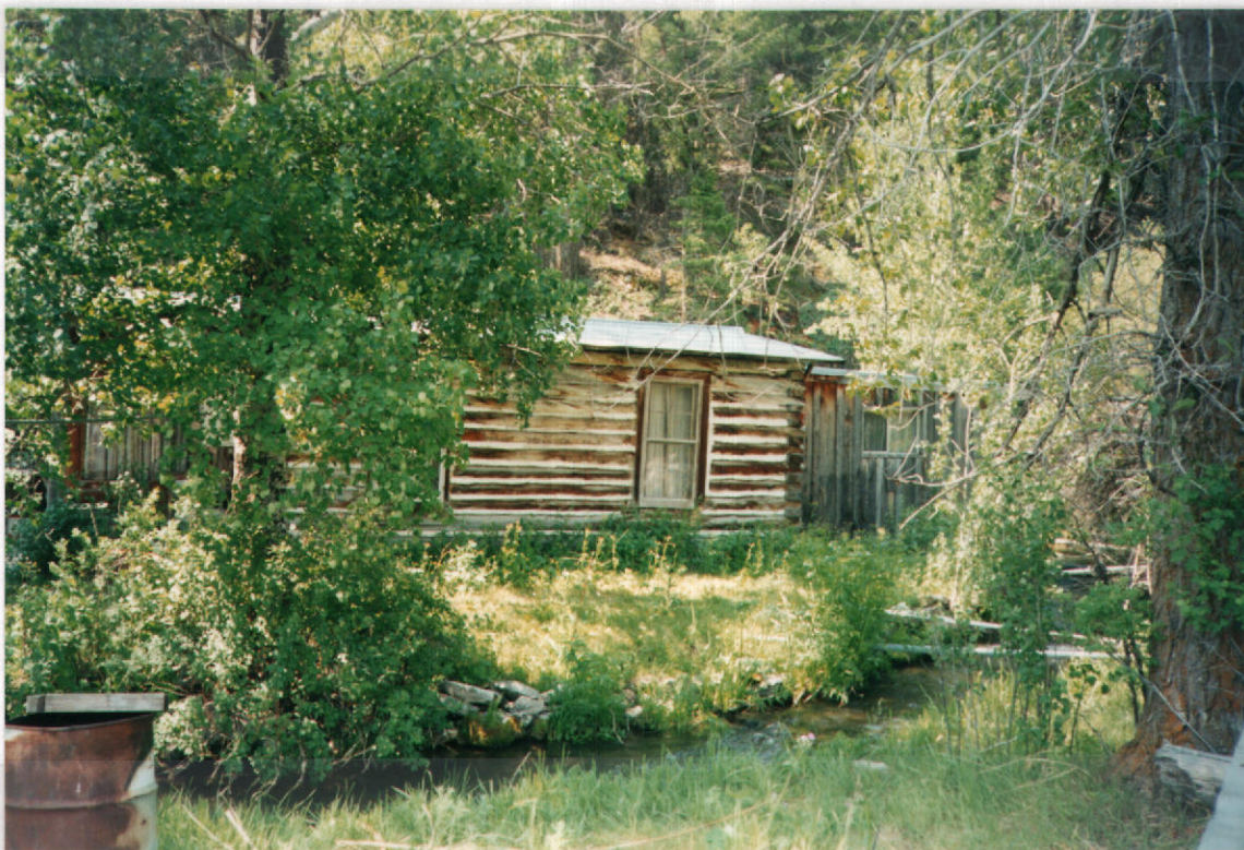
Fig. 8 - Cabin at place of use supplied by hydropower.
