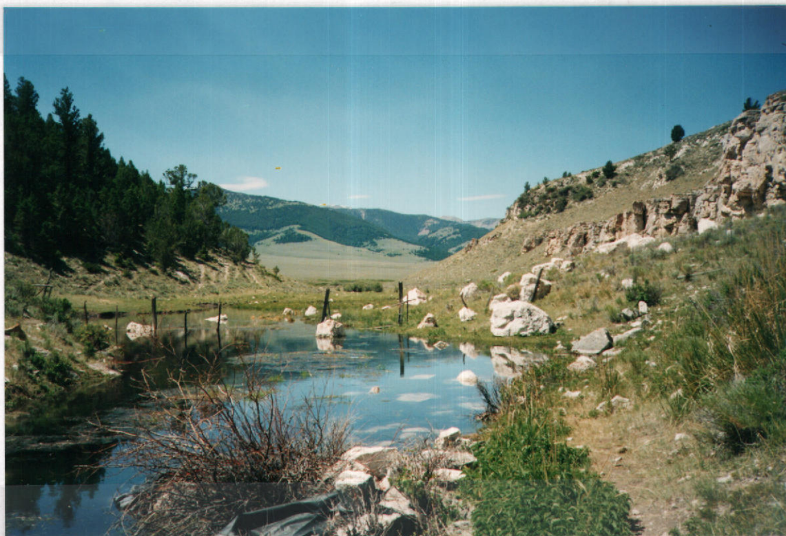
Fig. 2 - Fritz Creek looking upstream from diversion dam.
