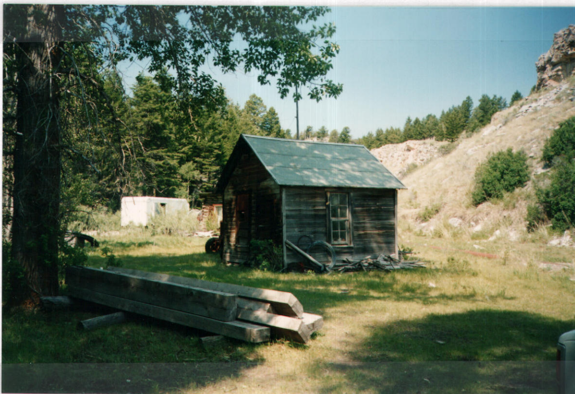
Fig. 9 - Shop building supplied by hydropower.
