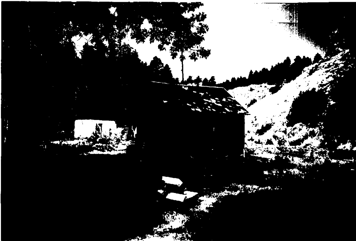
Fig. 9 - Shop building supplied by hydropower.
