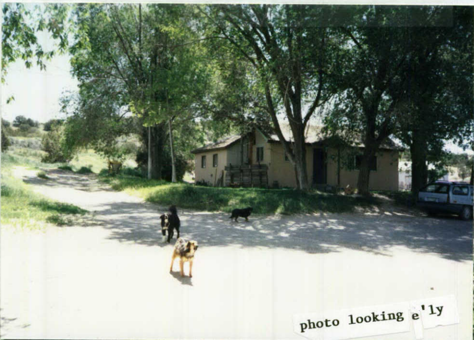
pump house here
