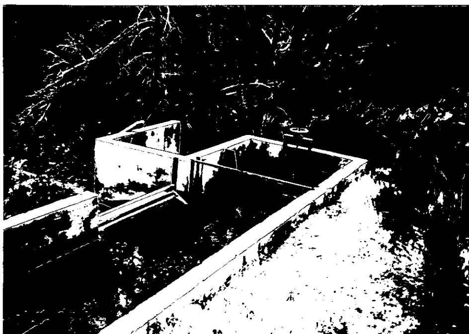
Diversion weir and overflow gate.
