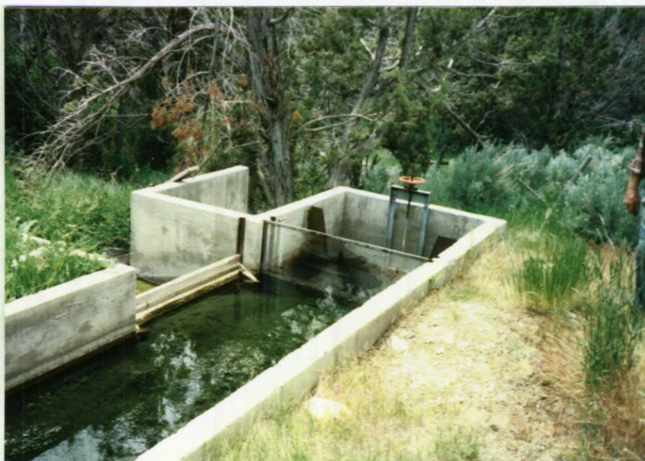
Diversion weir and overflow gate.
