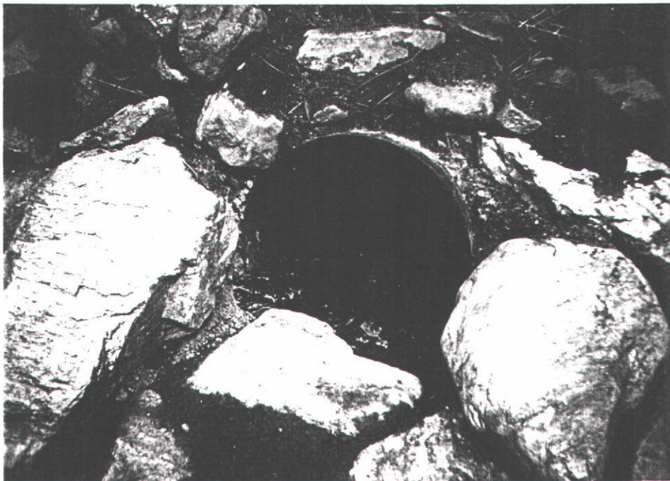
View of the intake to the 18" steel pipe that serves as the outlet/spillway for the reservoir.
