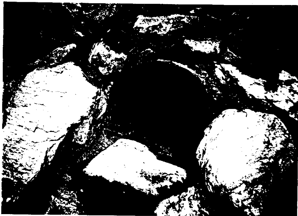
View of the intake to the 18" steel pipe that serves as the outlet/spillway for the reservoir.
