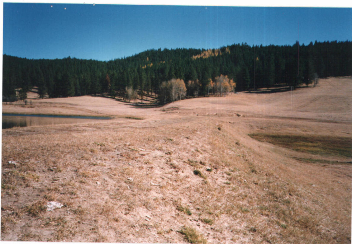
Looking east across point of diversion (dam) for reservoir.
