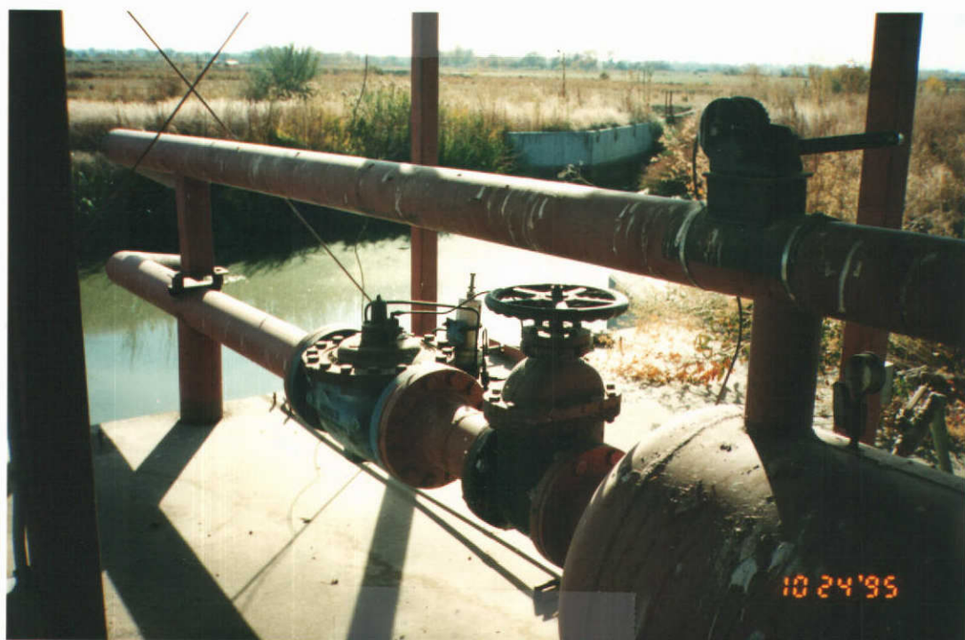
Inlet off of Lower Payette Ditch and Settling Pond
