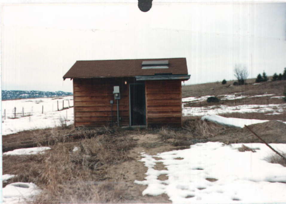
PUMP HOUSE LOOKING WEST
