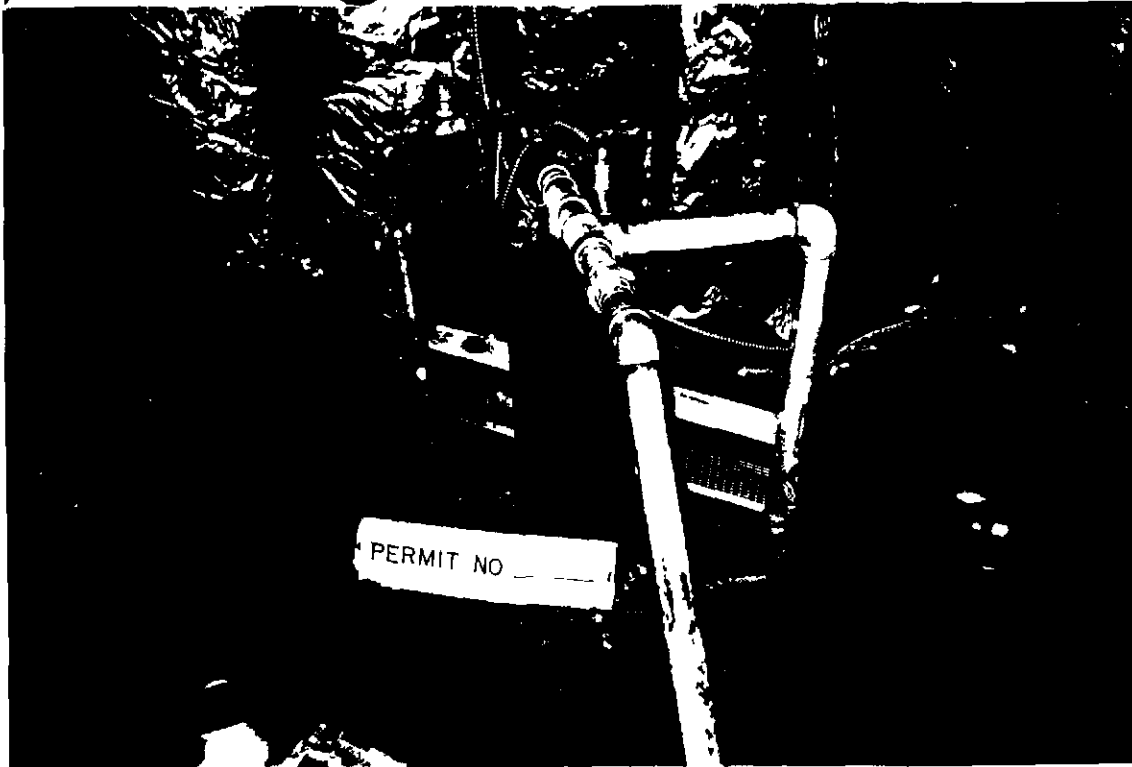
PHOTO ONE- Well in pump house. Site is near Eightmile Creek northeast of Lorman.
