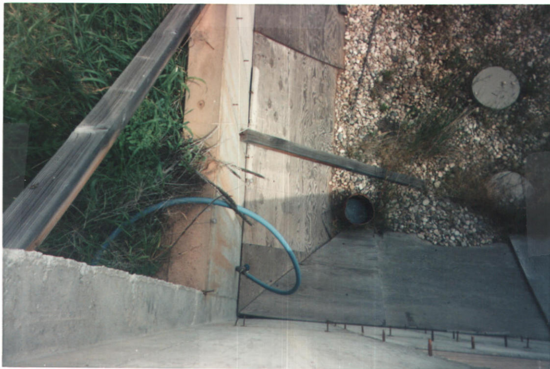
Hose with Faucet inside Foundation
