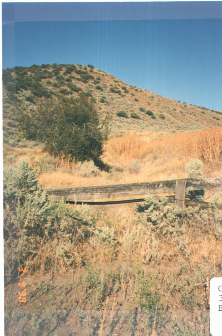
From the stockwater tank Number 1., Lookly North westerly. P/O approx. 100yds. Estimate from new owner. Pipes are all buried.
