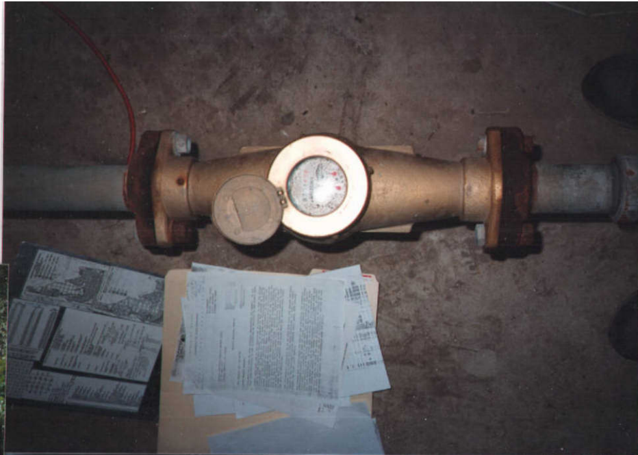
② Flowmeter in 2" pipe in well #1.
