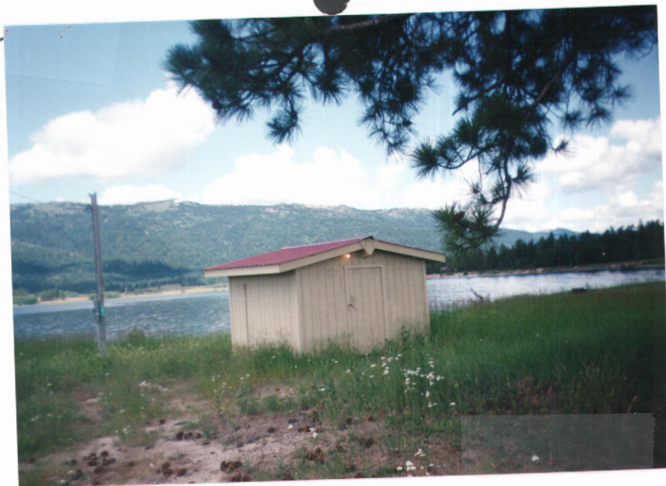
VIEW OF PUMPHOUSE THAT SURROUNDS THE PRESSURE TANK. THIS TANK IS THE ONLY TANK FOR THE WHOLE SYSTEM. CASCADE RES. IS IN THE BACKGROUND. THE WELL IS LOCATED TO THE RIGHT OF THIS SHED.
