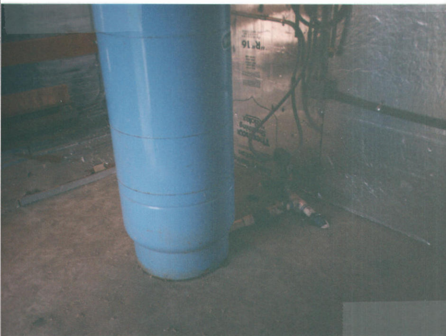
PHOTO THREE- View of the Pressure Tank & Lines that lead to the Domestic Hookups. Hookup Lines have been placed in locations for future Domestic sites.
