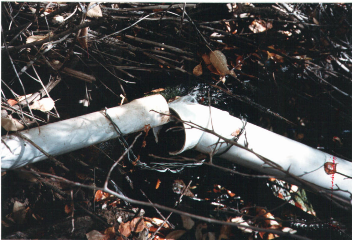
Measurement was conducted at this pipe
