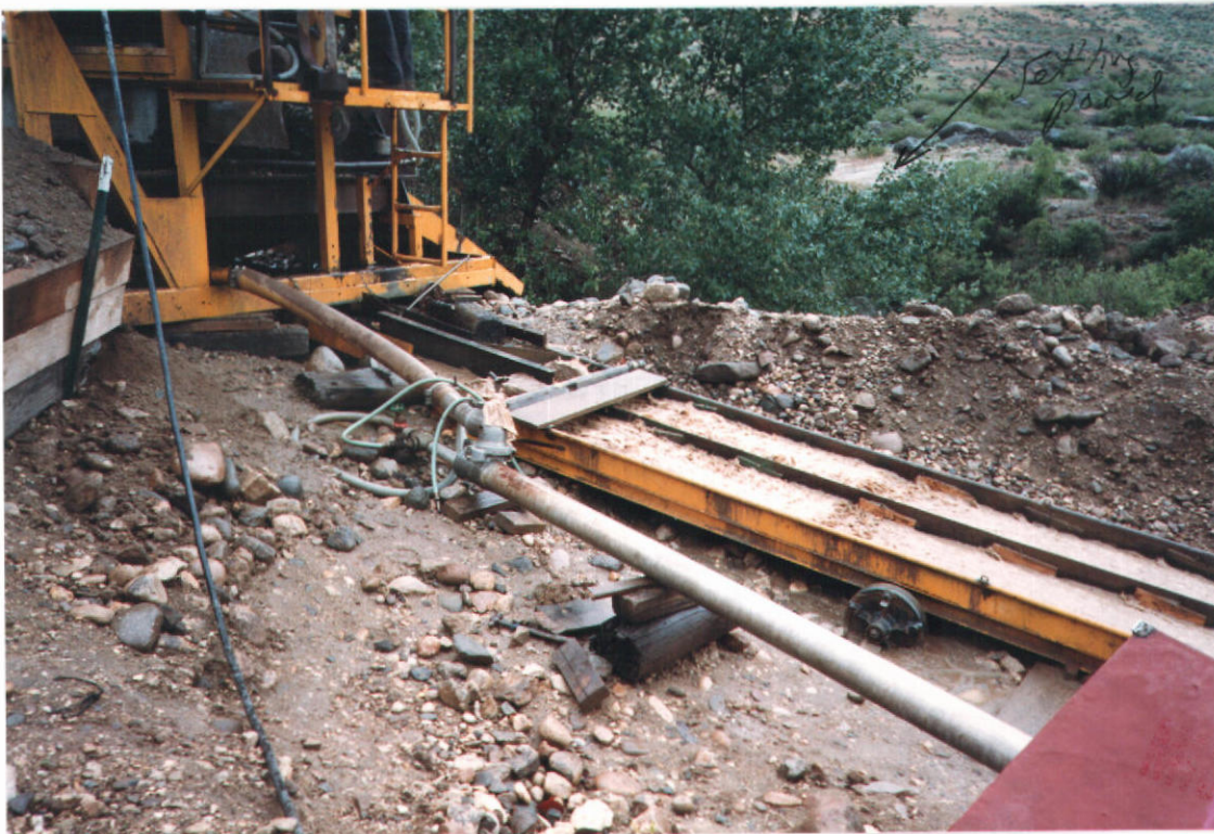
PHOTO TWO- Plus, typical operation on site. Note small settling pond in background. Several are found on site.
