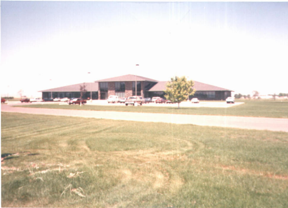
#5. P14 - commercial office building
