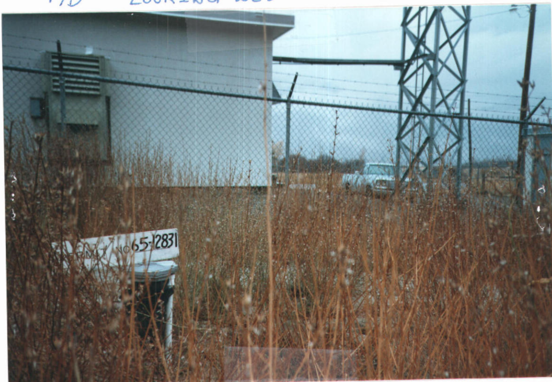
P/D LOOKING WEST
