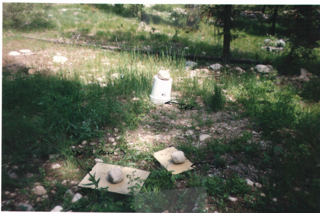
PHOTO FOUR- Irrigation and domestic valve boxes.
