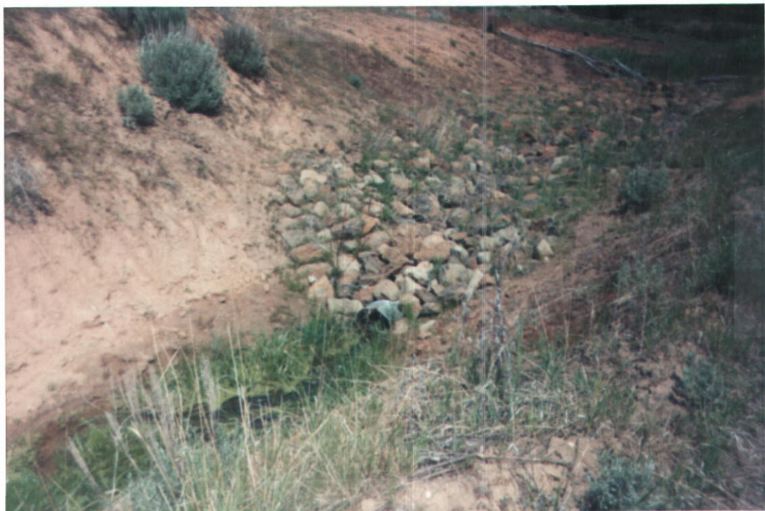
10" pipe leading from drain
