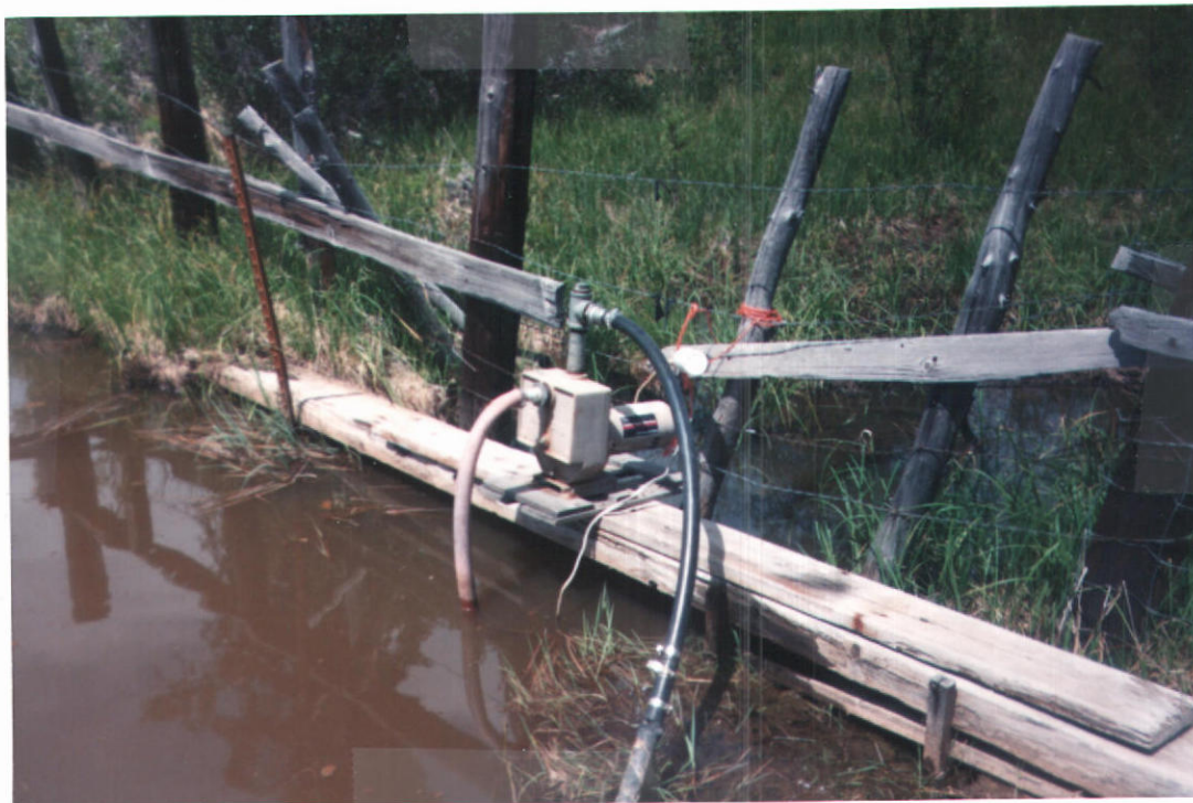
Pump #1 Ditch enters on right.
