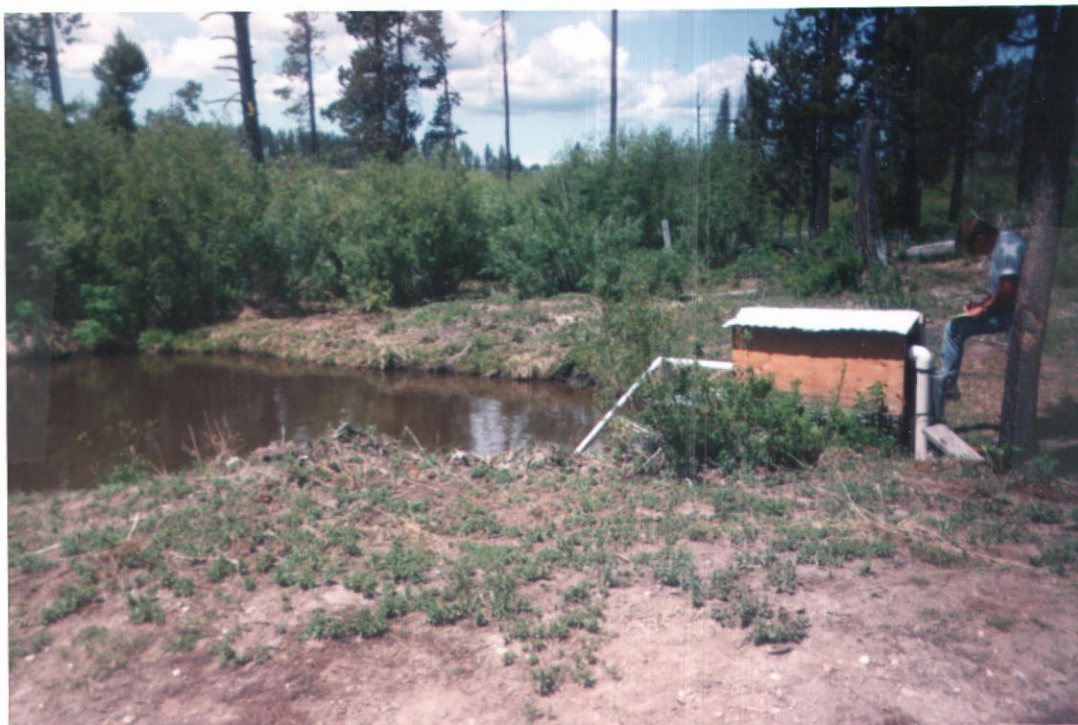
Pond #2. Facing Northwest
