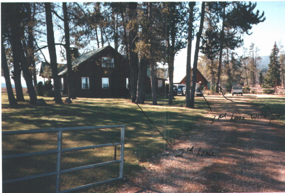
PHOTO FOUR- P/W, 2 other homes between RR tracks & Brush creek. View is SW. Yards here are irrigated with Brush ck. water (65-06628).
