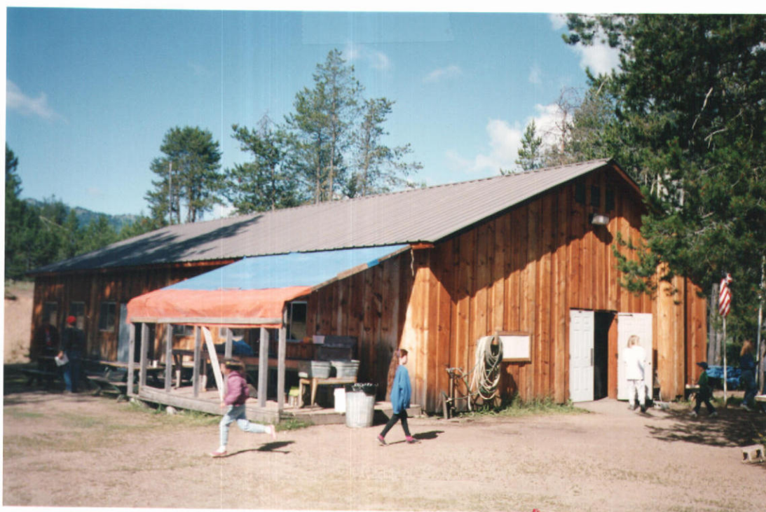
PHOTO FOUR- Kitchen and Dining Area Building
