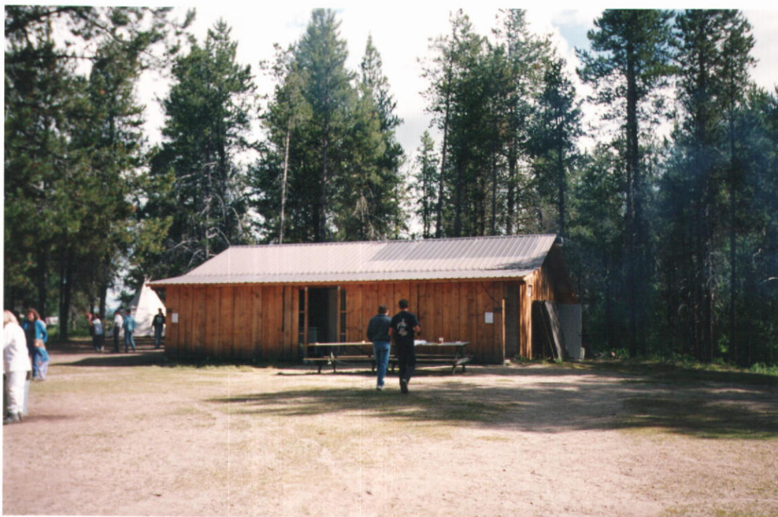
PHOTO THREE- Restrooms, Showers, and Laundry Building.
