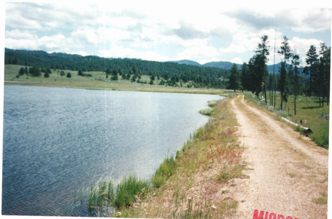
PHOTO FOUR- View easterly of south end of pond and dam.
