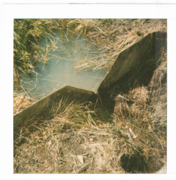
Upstream V Notch Weir
