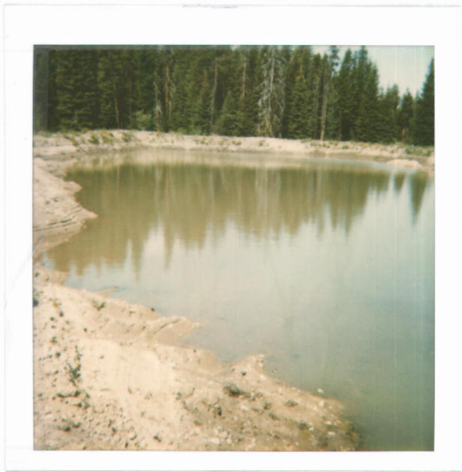
Reservoir and Dam
