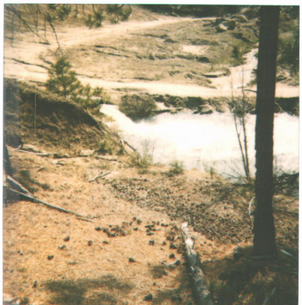
DISCHARGE PIPING TOM J DAM 65-13019 4/26/96
