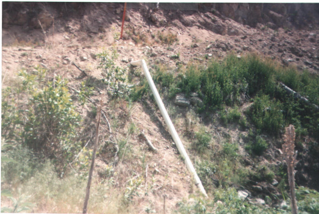
4" Overflow are west of storage tank.
