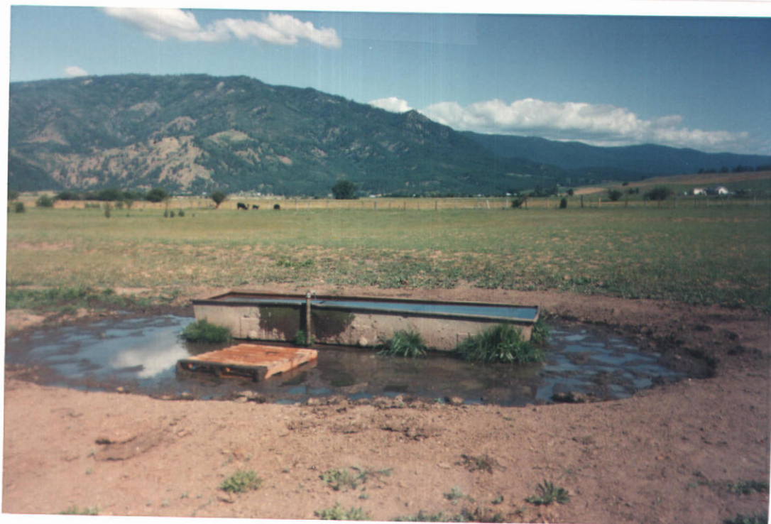
View Looking NW to 3' x 15' water Trough. Overflow on west end of Trough.
