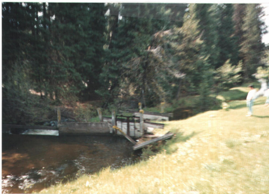
#6. Diversion dam on Boulder Creek where the Boulder ditch begins. This site is 4-5 miles North from the places of use.
