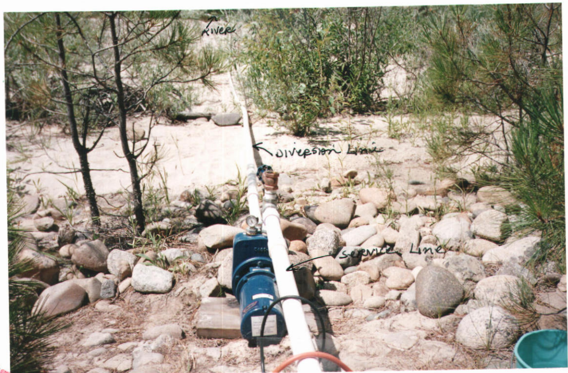
PHOTO ONE- Point of diversion in South Fork of Payette River. A portion of the approximately 175' of 2" PVC to pump on upper portion of river bank is shown.
