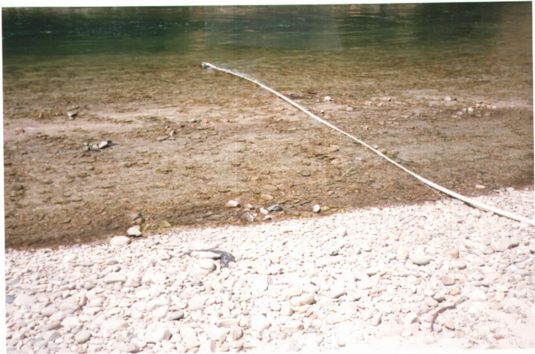
PHOTO ONE- Point of diversion in South Fork of Payette River. A portion of the approximately 175' of 2" PVC to pump on upper portion of river bank is shown.
