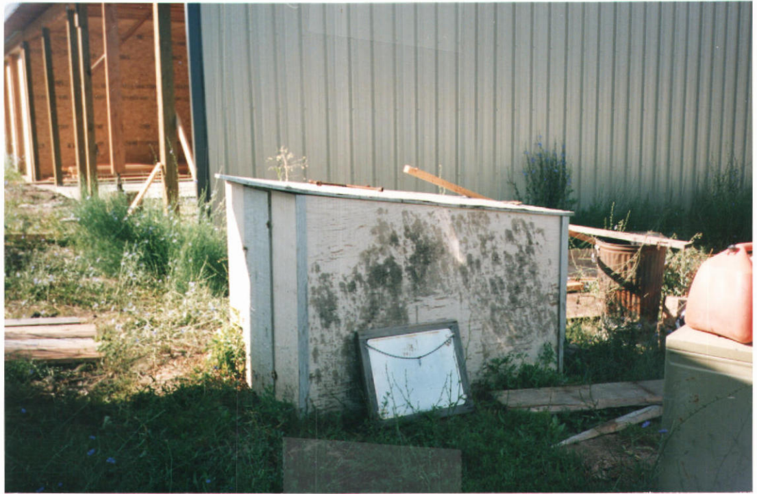
PHOTO ONE- Well house located near back of property.
