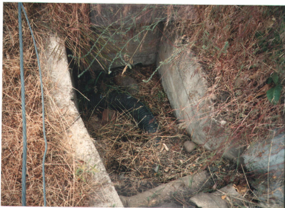
#4 Pipe carrying over flow under the road.
