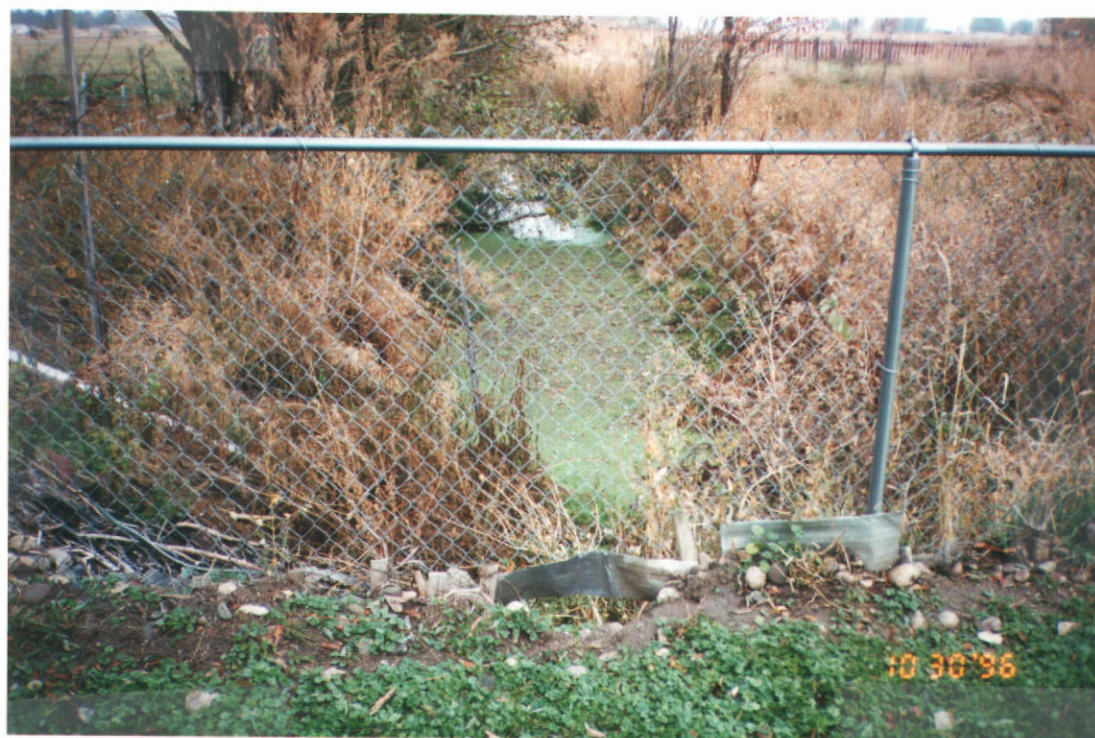
View Looking North.
